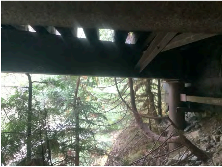
Right downstream flair girder
