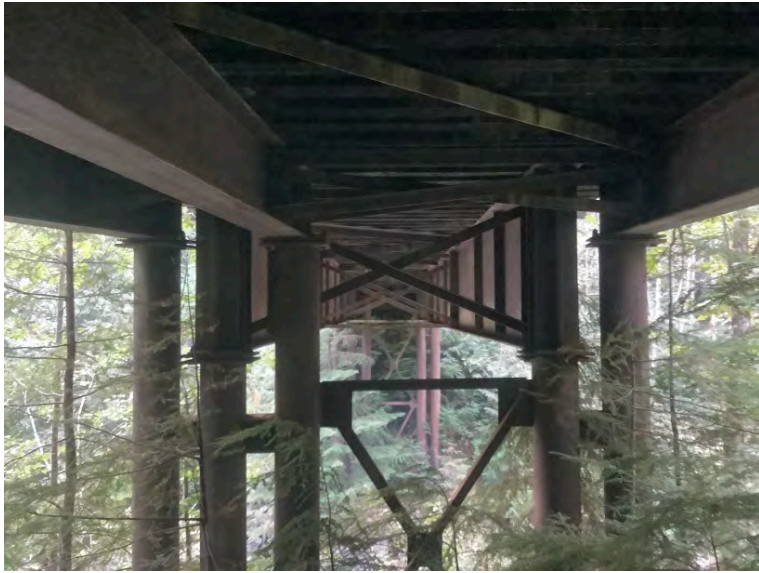
Span 2-3 pier viewing from left bank
