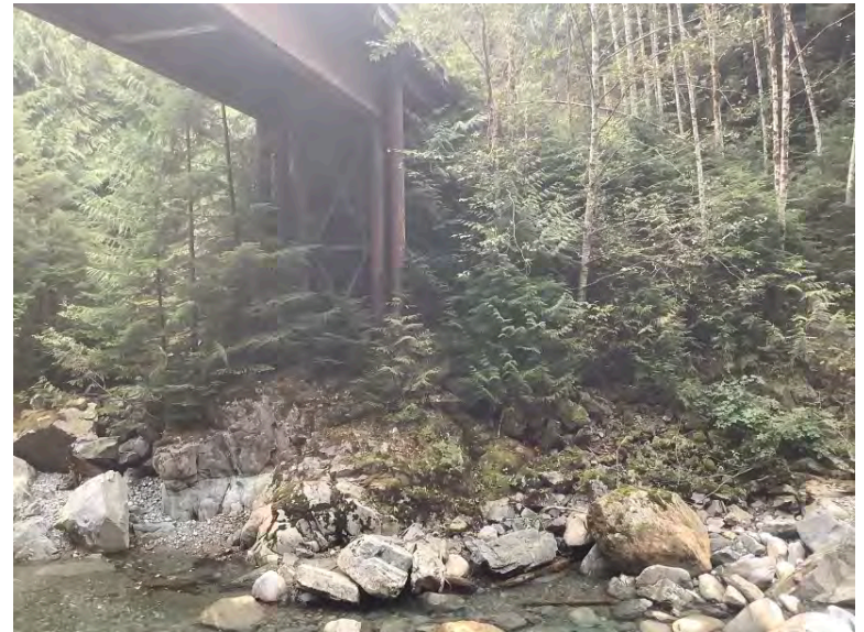
Right Bank Abutment when facing downstream
