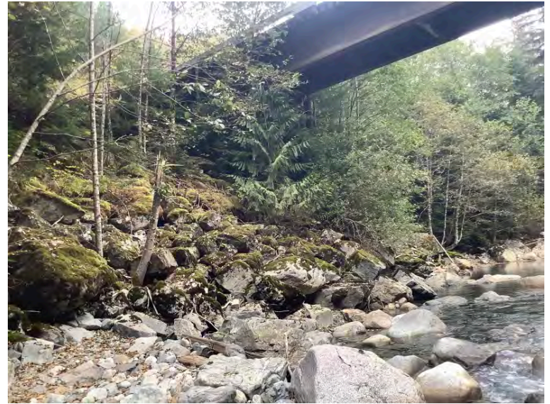
Left Bank Abutment when facing downstream
